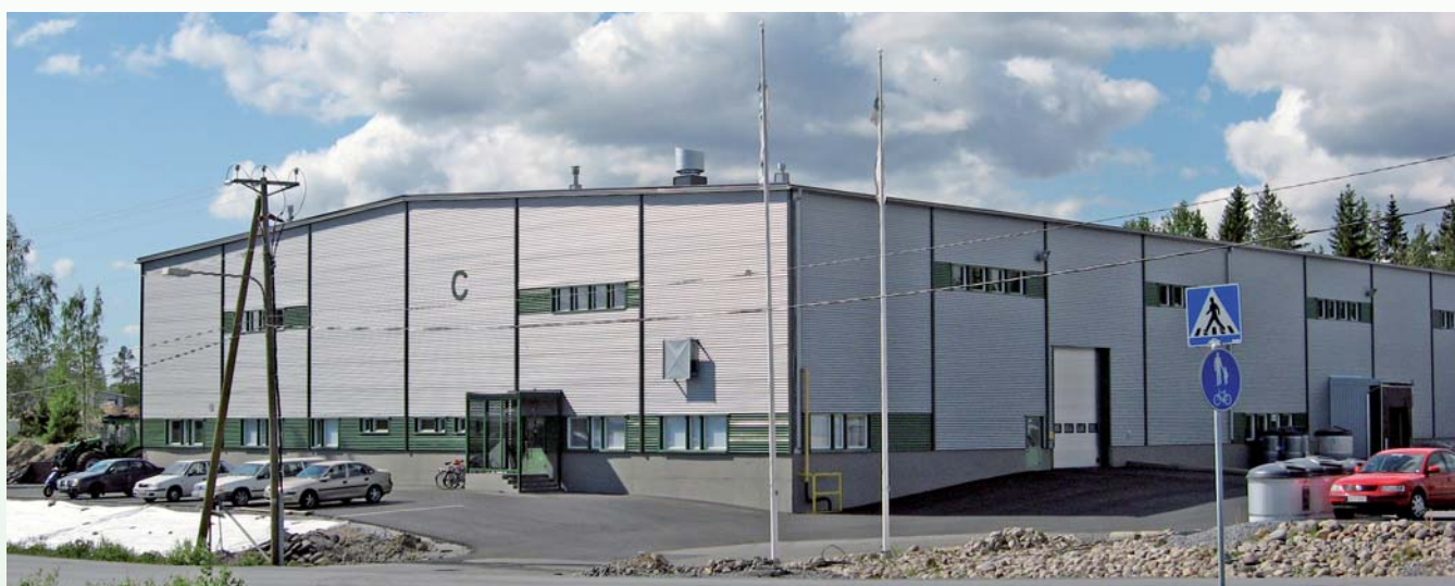
Molok's new factory expansion was completed in spring 2008.
